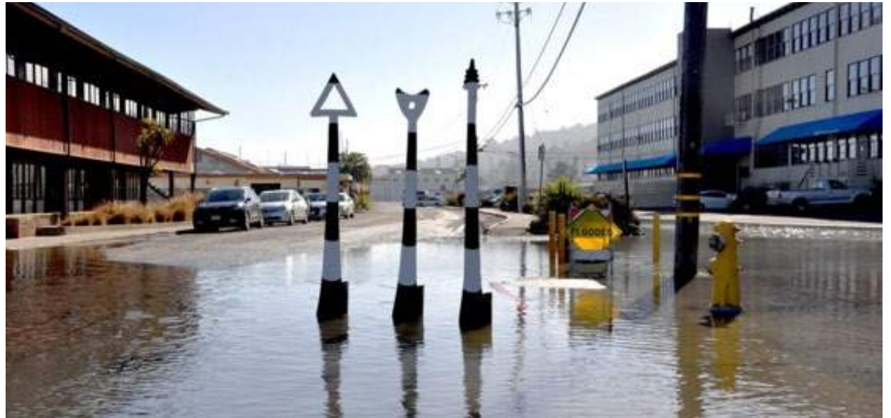
Flooding of Public Roads
